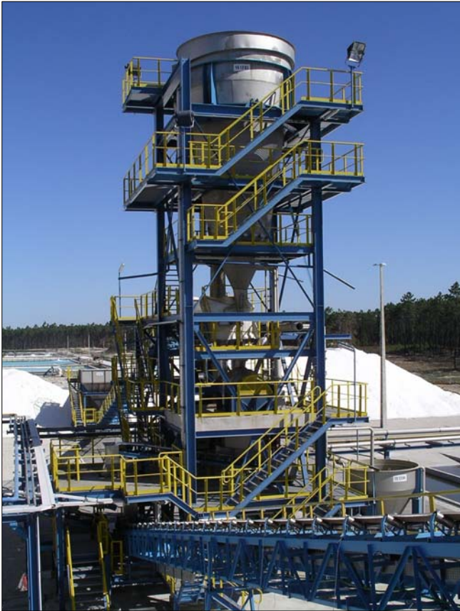
Renoeste salt upgrading plant with Hydrex-3 hydroextractor co-invented by Vladimir M. Sedivy, CH Patent No. 690840
